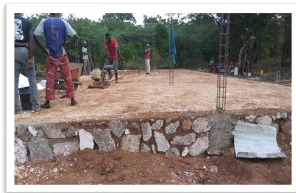
Chicken coop under construction
